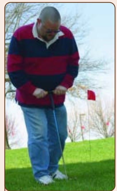
Figure 5 Probing for Trench Location
