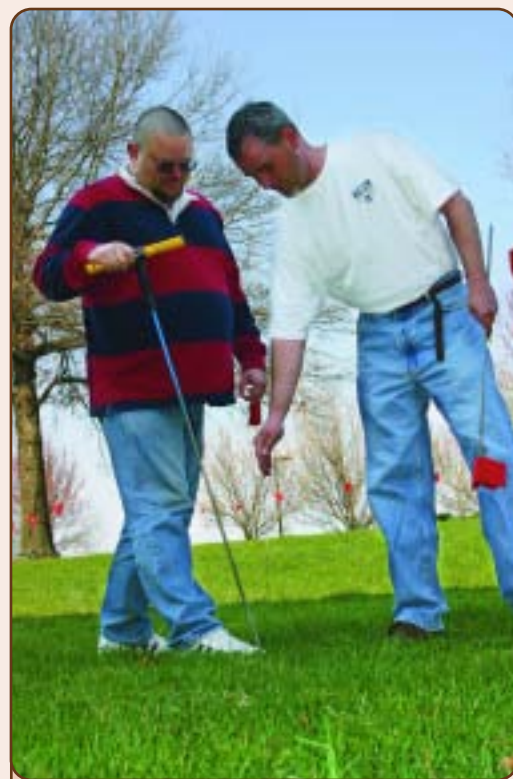
Figure 1 Identifying and Flagging the Drainfield
