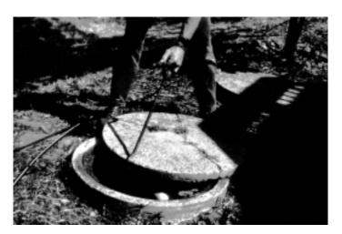
All mound systems at Auburn Lake Trails have tank risers, lateral valves and risers, inspection ports and groundwater monitoring wells. The management entity replaces trench monitoring risers and caps, flushes disposal bed lines, helps homeowners with advice on problem solving (odors, pump alarms, pumping) and performs legally required environmental monitoring.
