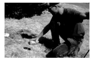
About 107 mound systems are inspected each year at Auburn Lake Trails. By catching problems early, they can be corrected by the management entity and reduce the environmental and public health impact. If a problem, such as ponding in the gravel bed, is identified the system is checked every three months to ensure that raw sewage does not come to the surface.
